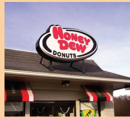
Roof Mounted Signs
