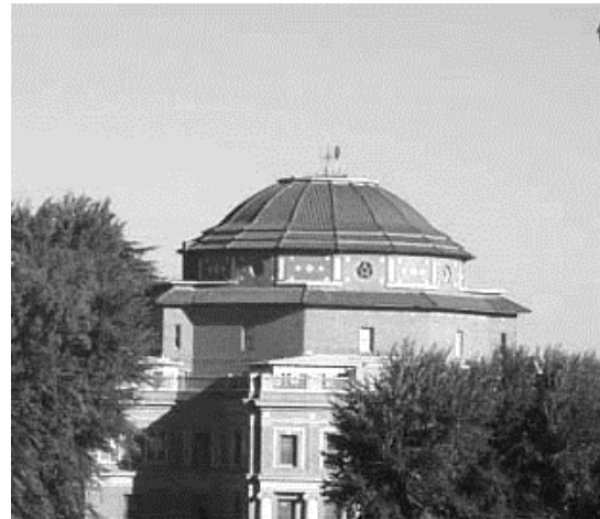
Photo 2. City Administration Building.
