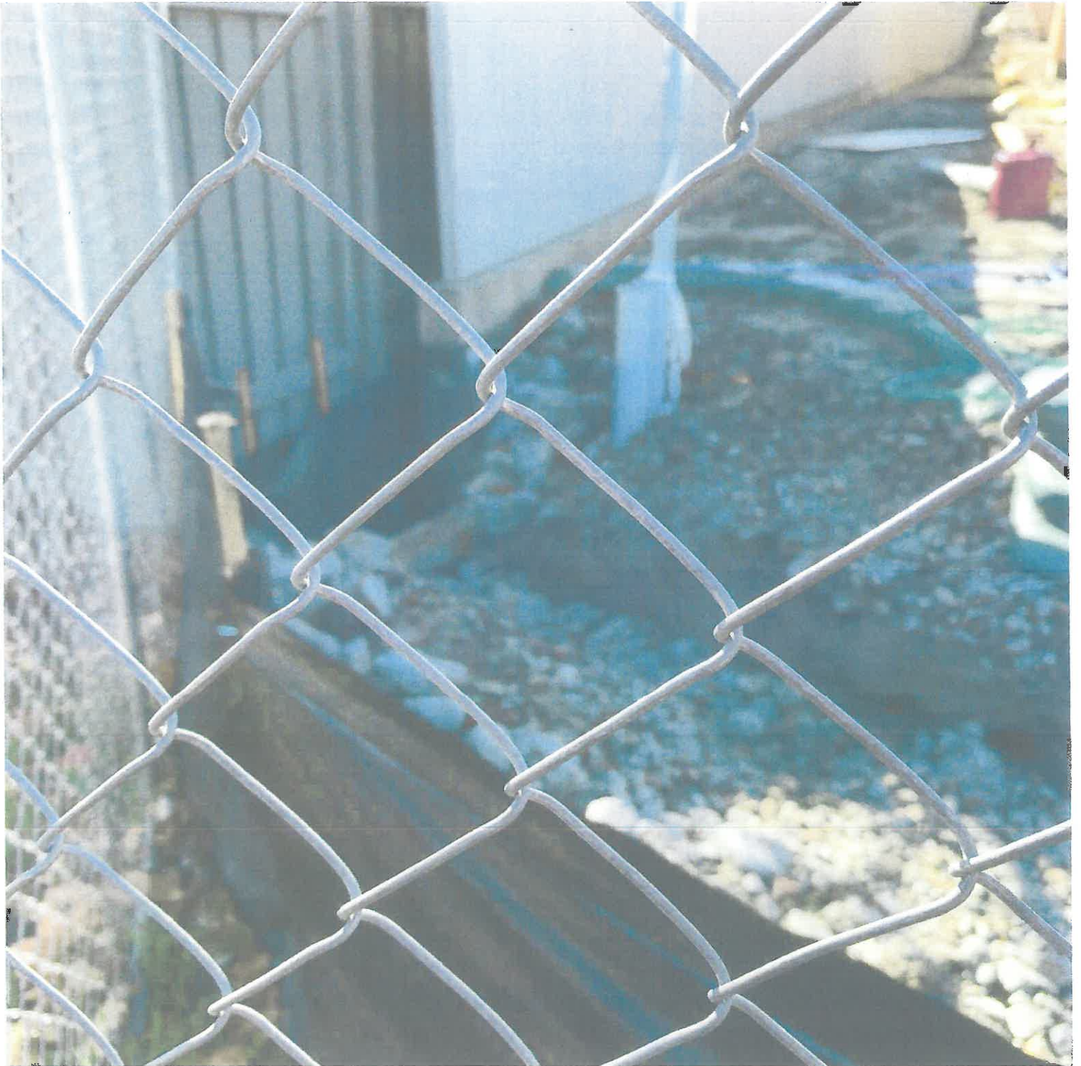
TRENCH LEADING TO CHANNEL BEHIND 900 AND 910 LA COSTA COURT
