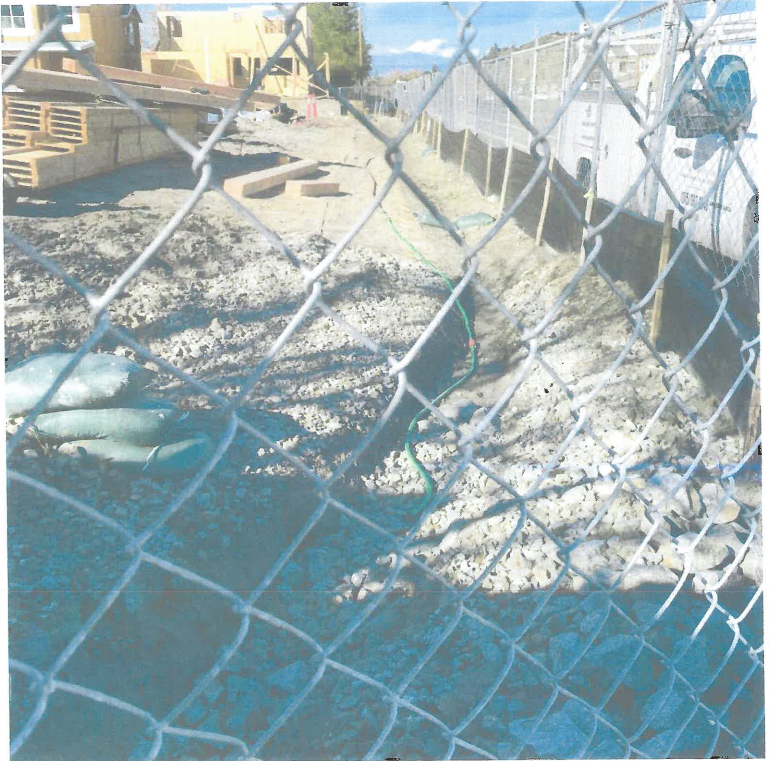
TRENCH ALONG EL CAMINO REAL
