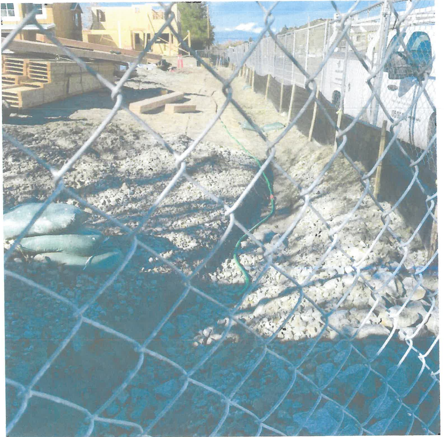
TRENCH ALONG EL CAMINO REAL
